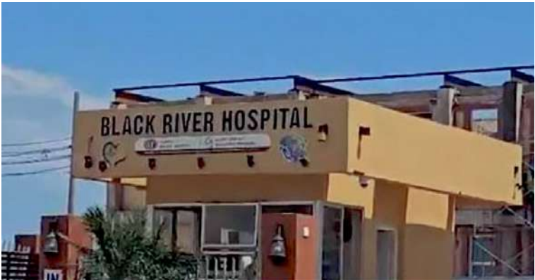
Reconstruction works at the hurricane-damaged Black River Hospital in St. Elizabeth.
