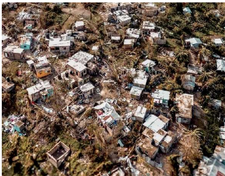
Houses and hotels were damaged particularly in the southwestern side of Jamaica. (Facebook image)
