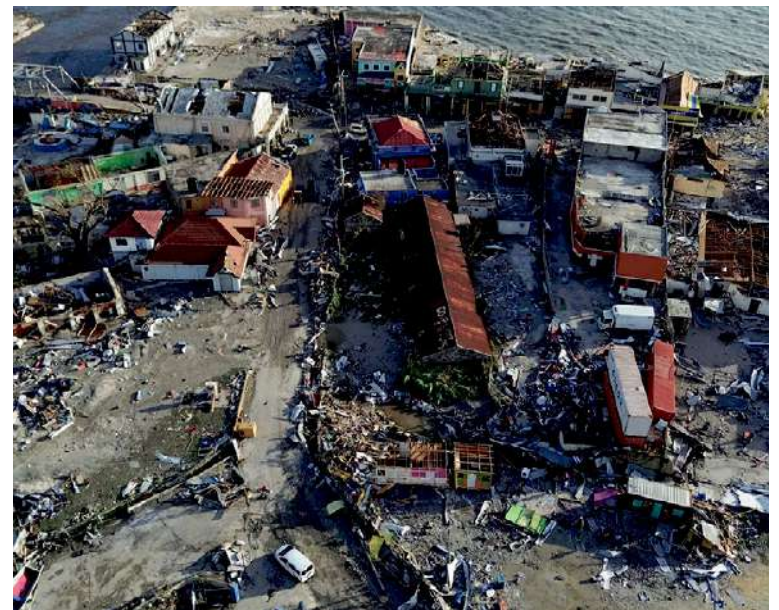
Drone footage shows the damage in Blackriver, St. Elizabeth. (Getty image)
