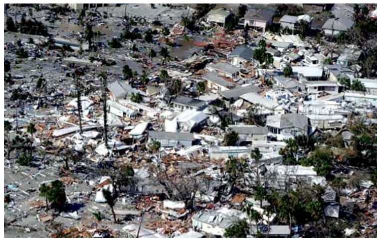
Damaged homes and debris are shown in the aftermath of Hurricane Ian in Fort Myers, Fla. on Sept. 29. (Photo: AP Photo/Wilfredo Lee)
